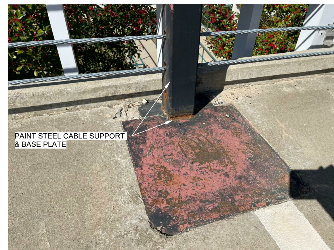
45.10 PAINT STEEL CABLE SUPPORT & BASE PLATE
