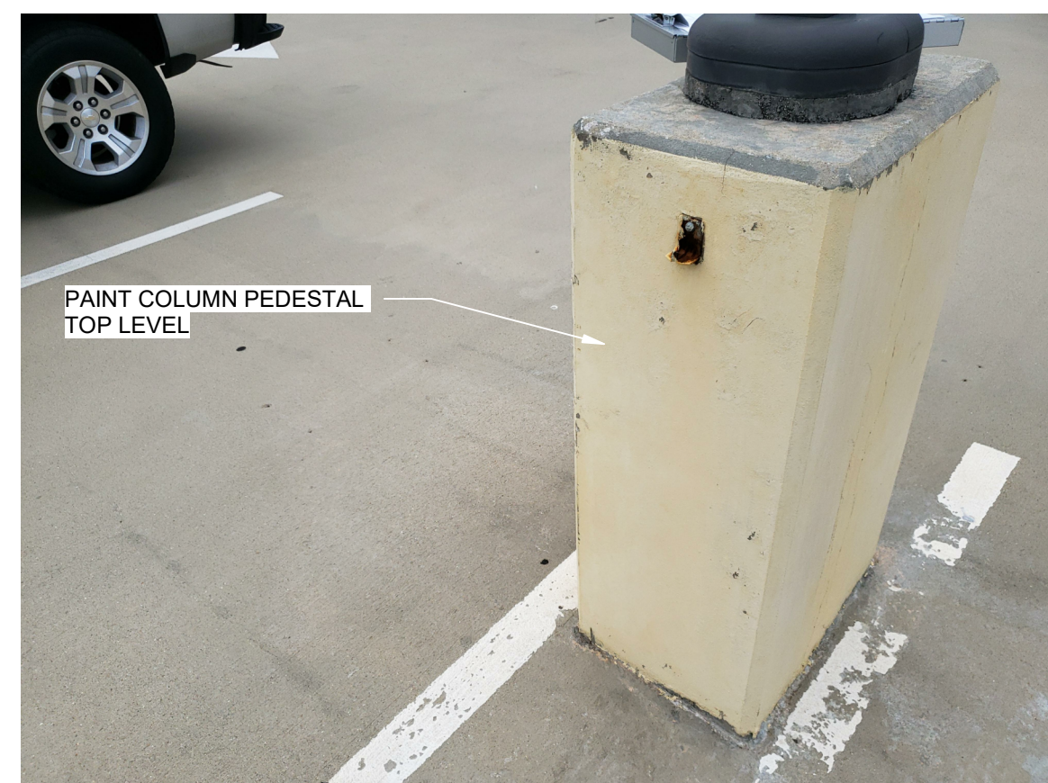
45.9 PAINT COLUMN PEDESTAL TOP LEVEL
