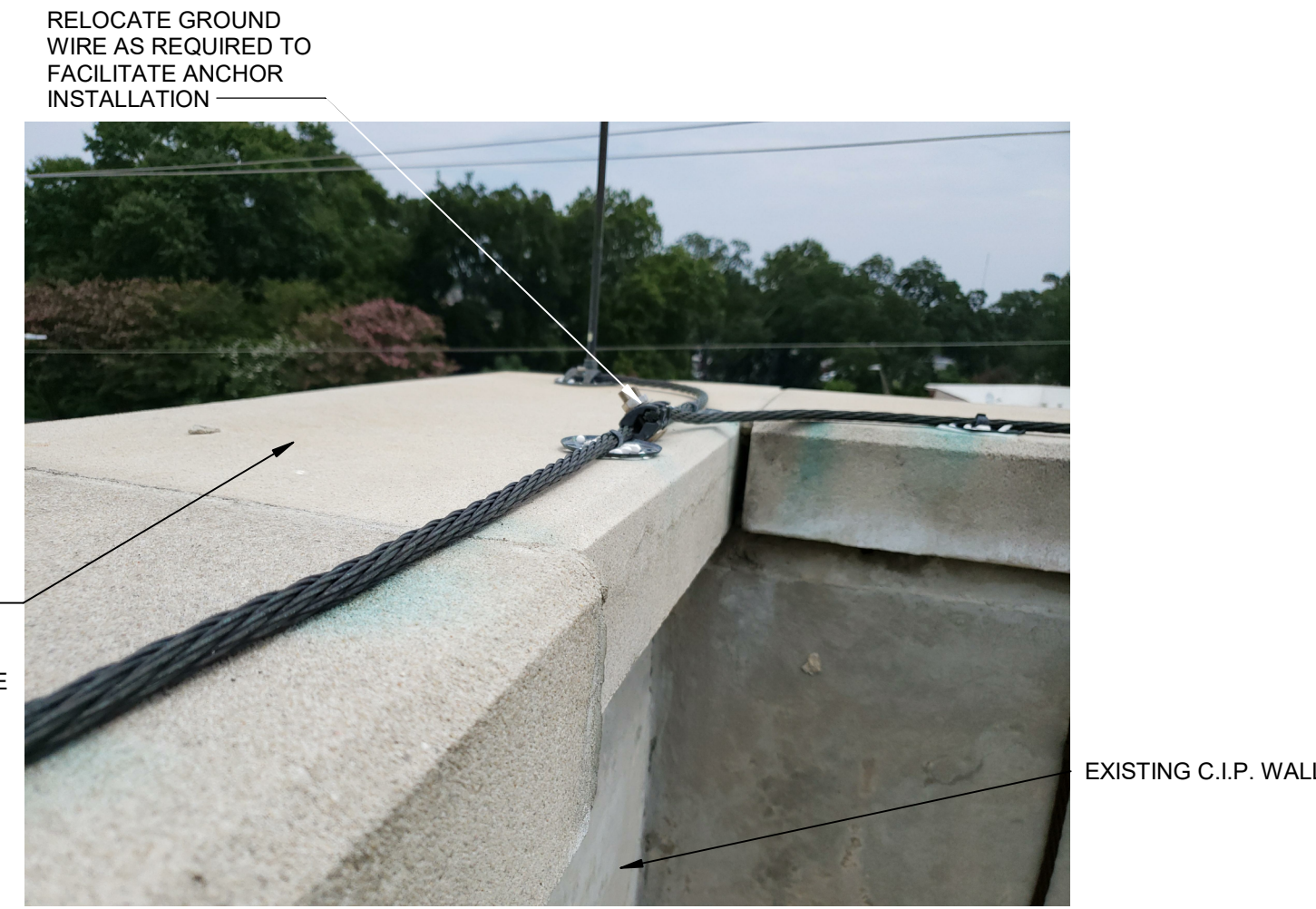
2 EXISTING CORNER CONDITION (PHOTO)
