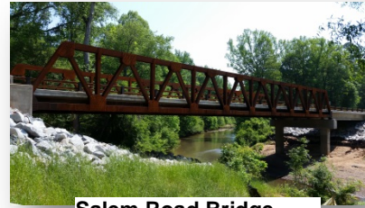
Salem Road Bridge
