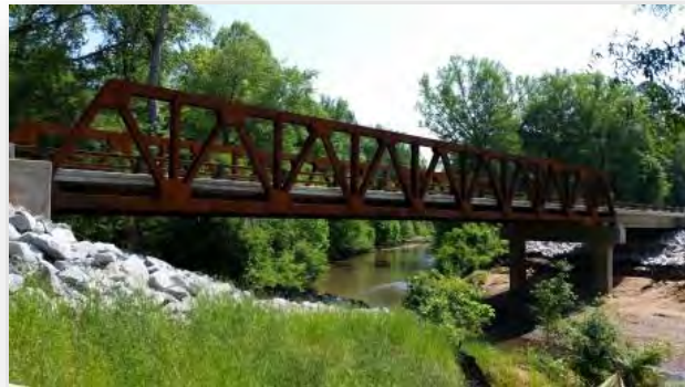
Salem Road Bridge
